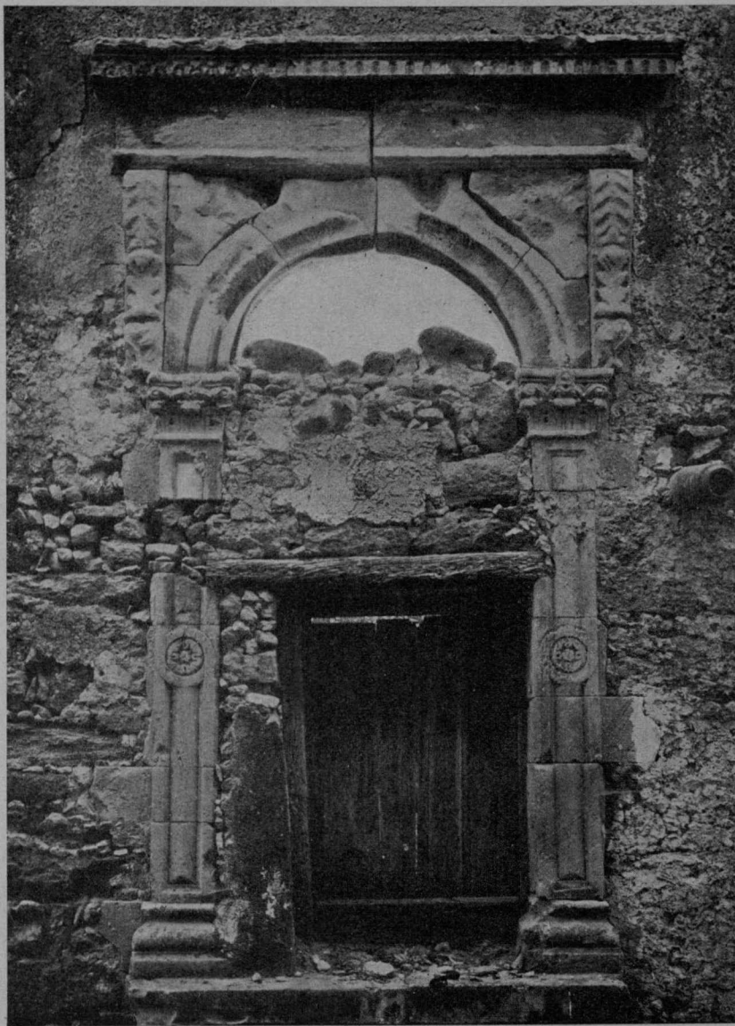
FIG. 137 — RETIMO — FINESTRONE IN VIA PREVELL. (377).
